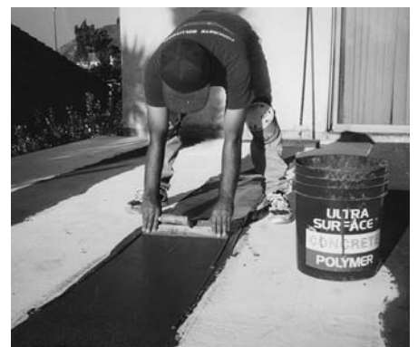
If applying a thin coating system over the fabric it will be necessary to first patch the seams with Ultra Surface Polymer Concrete using a trowel or metal squeegee and then to apply a Squeegee/Bond Coat over the whole surface.
