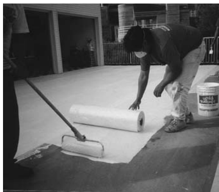
Roll The Fabric into the wet Elastomeric Basecoat a few feet at a time.
