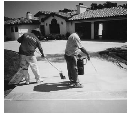
Apply Colorcoat 100 diluted with 1-2 parts of water using a sprayer and a soft broom. When dry apply a topcoat of Sealcoat 1000 clear.
