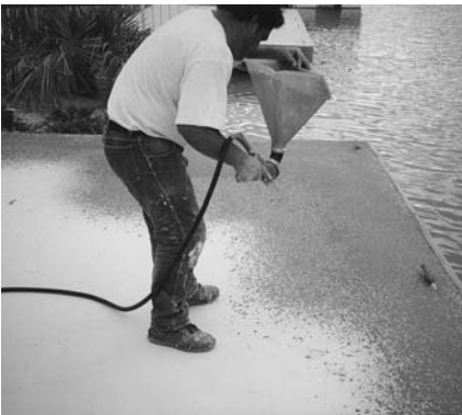
Spray the Ultra Surface Trowel Knockdown Mix using a hopper gun sprayer.
