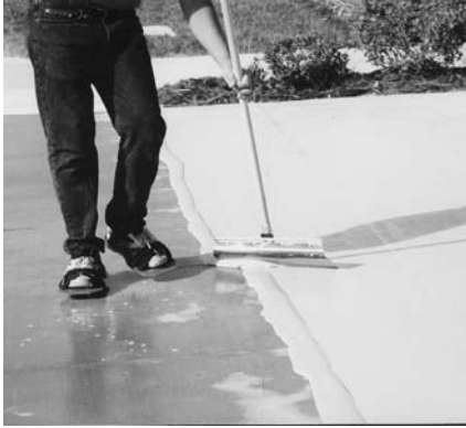
Apply a Squeeze/Bond Coat of Ultra Surface Polymer Concrete over the surface.
