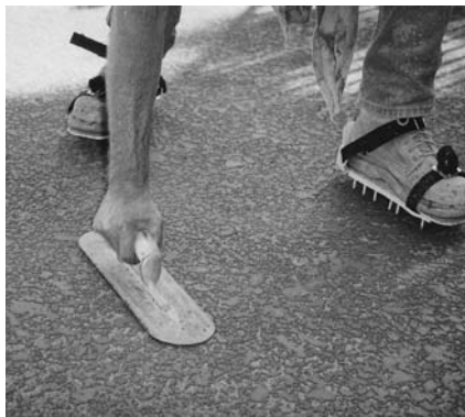
Trowel the sprayed Trowel Knockdown Mix to achieve the desired texture.
