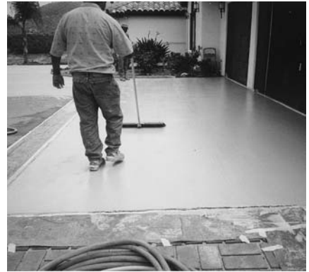
Option: Apply a Texture Coat after the first Squeegee Coat dries.
