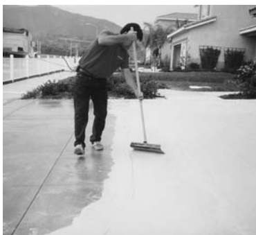
Spread the mix from side to side, in straight rows using a special metal edge squeegee.
