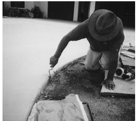
Scrape or brush the vertical edges where the material drips over the sides.
